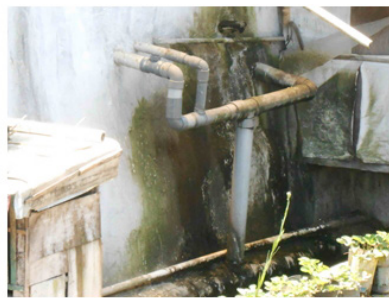
Figure 10. Private water well, powered by electrical pumping Source: Private Collection, 2015
