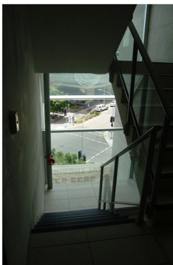
Figure 8. Case 4 Stairwell with natural ventilation and daylight Source: M. Kisluk.
