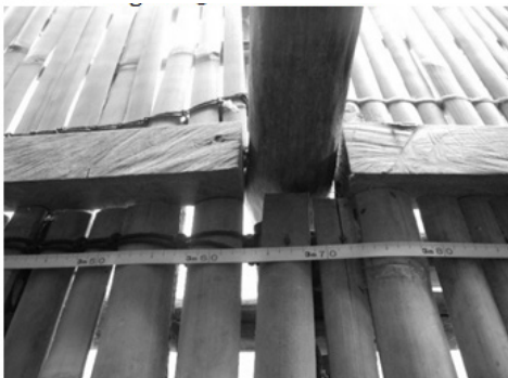
Figure 15. Typical bamboo floor
