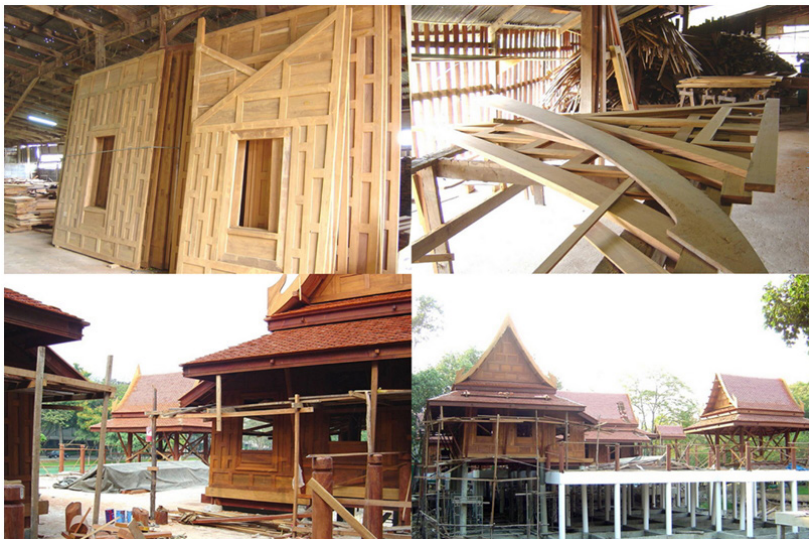
Figure 3. House panels in carpentry (top) and assembly on site (bottom) Source: (Nongnit's Treasures, 2011)
