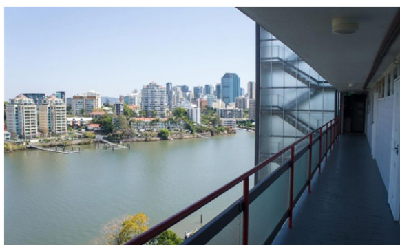
Figure 6. Case 1. View from gallery access corridor toward stairwell. Source: Image by M Fletcher, QUT.
