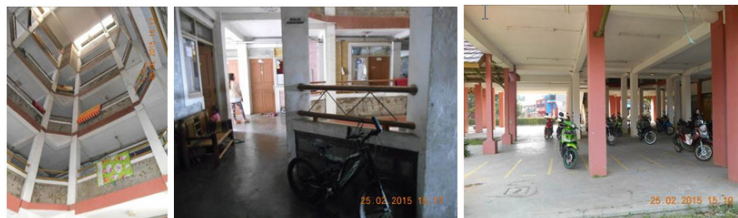
Figure 4. Cigugur Tengah flat building conditions Source: Authors' documentation
